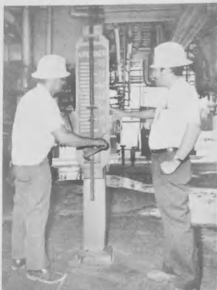
Adjusting the # 5 PS Crude furnace stack damper and observing the draft gauge reading are Eddy Laclé and R. Benjamin Lampe.
